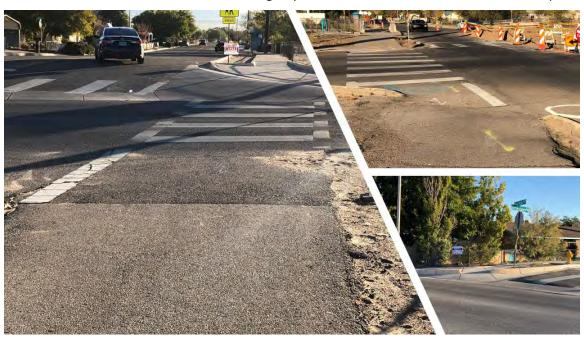
**Photo 2- Existing Non-ADA Compliant Curb Ramps**
